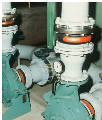
STENFLEX® type A-1 used at pumps
