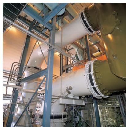
STENFLEX® type C-31 in a power plant
