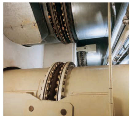
STENFLEX® type C-1 with special high restraints in cooling water system of a power plant
