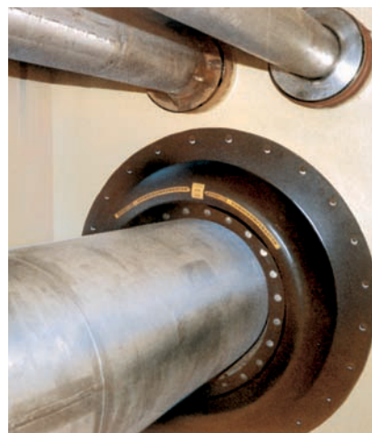
STENFLEX® type W-2 in a power plant
