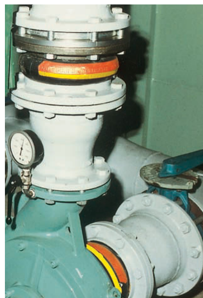
STENFLEX® type AR-1 used at pumps
