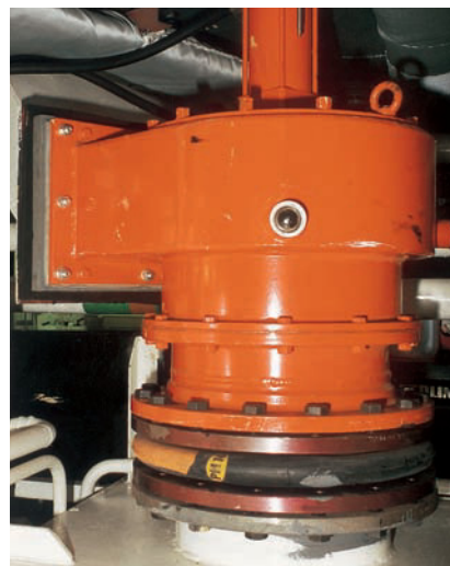
STENFLEX® type B-1 for compensating large movements
